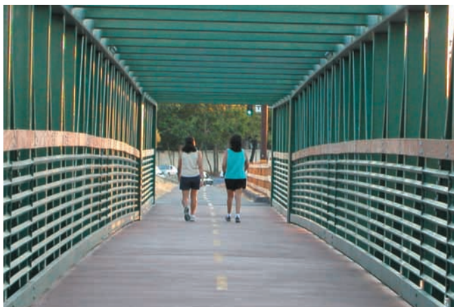
(003GuadalupeTrailBridge2.jpg) Bridge construction provides for span of the riparian corridor and adequate width for trail users.
