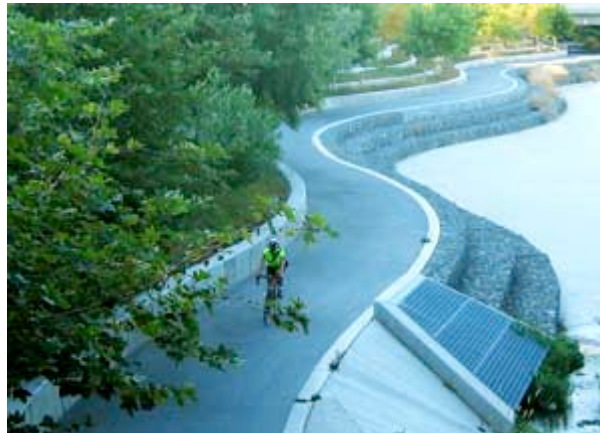
The trail system is built as part of the larger flood improvement process
